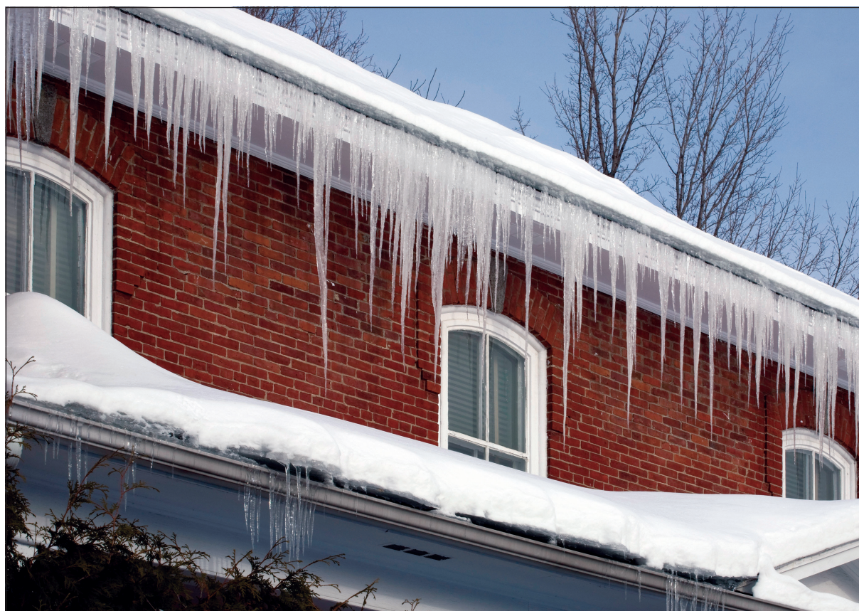
Frozen gutters can be the cause of a variety of winter home problems.
